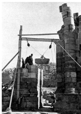
Above left: Petra is littered with fallen columns. Left and above: In 1962 archeologists began reconstruction work in Petra, lifting columns and walls back into place. In many cases they could easily tell how to do the reconstruction as the columns and walls lay completely on their sides. (The Illustrated London News, March 31, 1962, Page 502/503, Archeological Section no 2085, Used by permission.)
